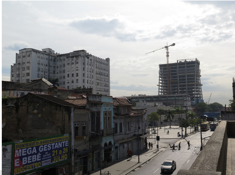
Figure 5: Early stage of construction of the new Porto Maravilha towers along the Camerino axis, near the Boulevard Olímpico. The immediate surroundings include architectural examples characteristic of distinct urbanization phases.
