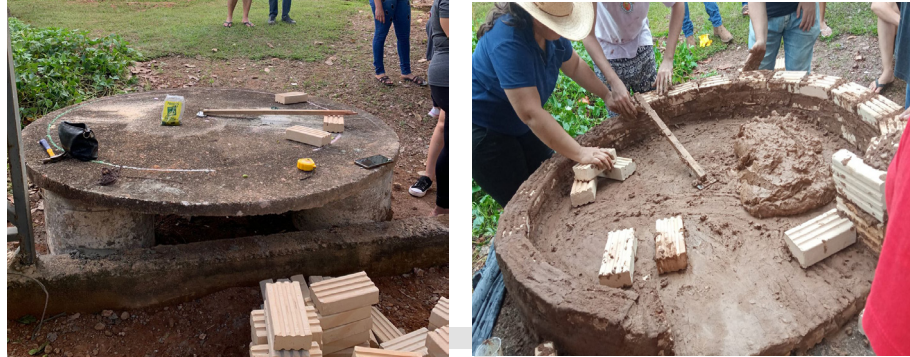
Figure 3: Marking and first rows of bricks.
