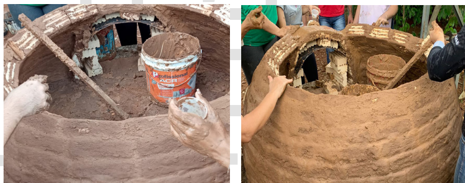
Figure 4: Brick laying.
