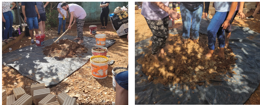
Figure 2: Mortar for brick laying. Source: Elaborated by the author, 2023.
