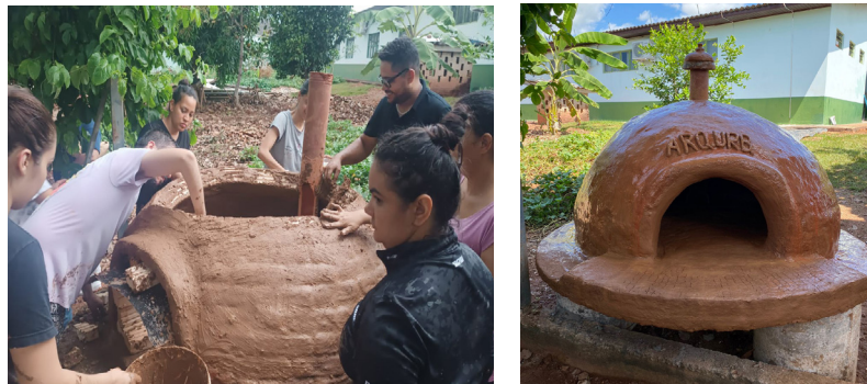
Figure 5: Final rows of bricks and completion.
