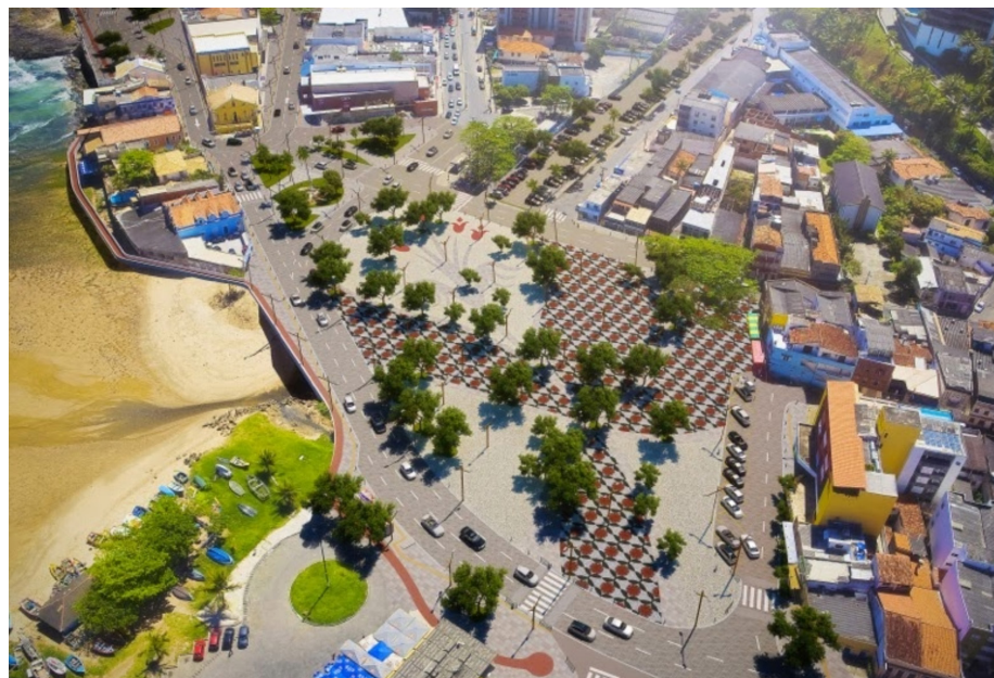
Figure 2: Promotional image of the project for Largo da Mariquita, published in February 2014. Available at: http://salvadoremumdia.blogspot.com.br/2014/02/apresentado-projeto-de-requalificacao.html . Access on: 2 Apr. 2017.
