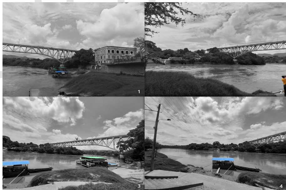
Figure 3: Table of images. Image 1: Perspective on the Magdalena River, El Embarcadero, and the Iron Bridge; Image 2: Perspective on the Magdalena River overlooking Flandes, Tolima; Image 3: Iron Bridge and boats on the Magdalena River; Image 4: Boat on the Magdalena River. Source: Lab-Strategy; FAUMack; Girardot, 2023.
