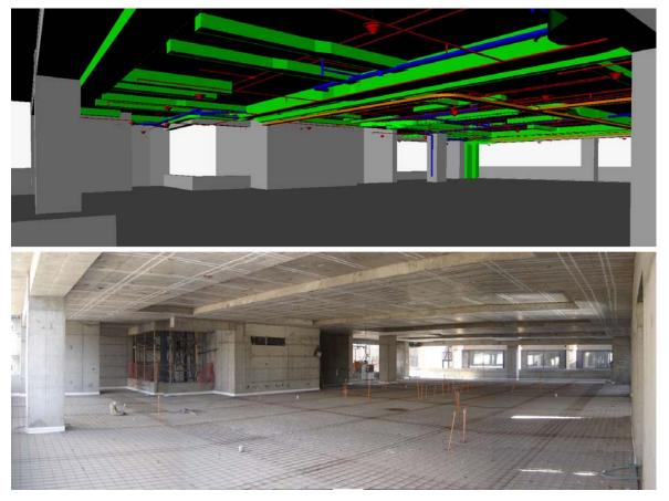
Figure 1: Job site image and coordinated BIM model developed by the firm Modelacion Digital from Chile (image courtesy of Modelacion Digital, Chile, 2008).
