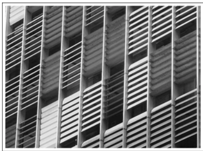
Figure 12 - South American Bank Building Detail of shading devices system on Northeast façade. (Photo by Rechilene Maia)
