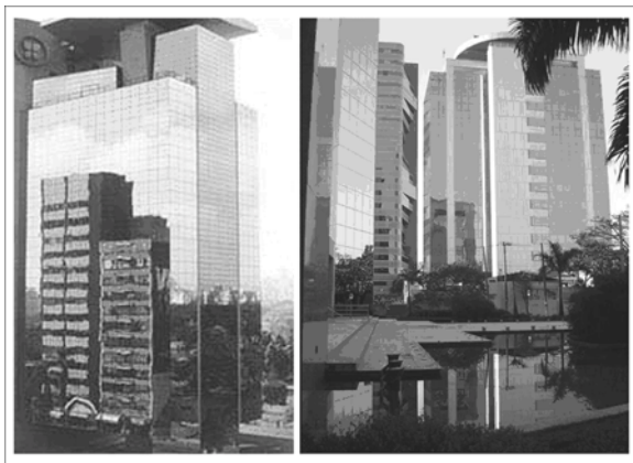
Figure 13 - Commercial buildings from 90's in São Paulo. (Images from Internet).
