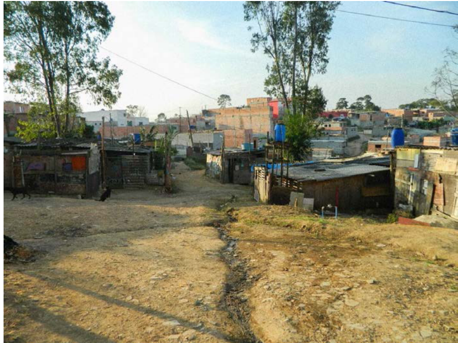
Figure 4: Drainage in the streets of Jardim Gaivotas, São Paulo. Used water flows into eroded cracks in the open. Source: João Gabriel de Oliveira (2022).
