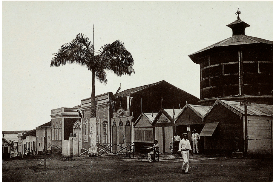
Figure 1: Water tower at Largo dos Remédios, Manaus (1884), demolished. Source: George Huebner / Instituto Moreira Salles Collection (public domain).
